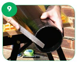
Ensure all the cut lengths of pipe are chamfered to roughly a 45 degree angle.
