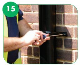
✓ Then using 40mm x 5.5mm roundhead brass or zinc screws, attach the first bracket to the pipe.
