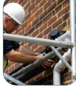
✓ For replacement, first remove the existing soil stack and fittings, starting at the top of the stack and working your way down.
