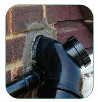
To complete the installation, use a cement mix to make good any holes.
