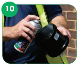
Use a silicone lubricant to make the fitting easier.
