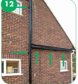
Fit the pipe or socket brackets at a maximum of 2 metres on vertical pipe and a maximum of 1 metre on horizontal pipe.
