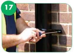
✓ Then measure and install the connecting branch and pipes securing with FloPlast's pipe or socket brackets.
