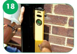
Ensure pipe is vertical by measuring with a spirit level.
