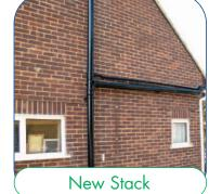
Install the new soil stack in the reverse order of the removal of the old stack working from the ground to the top. A brand new installation should also be carried out in this way.
